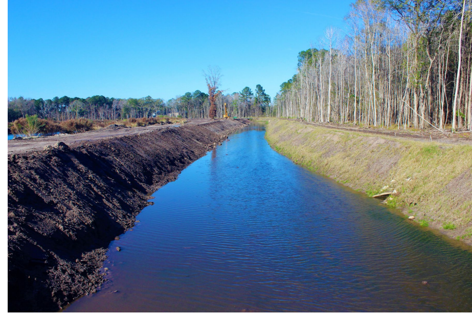
Improved section of Pipemakers Canal
