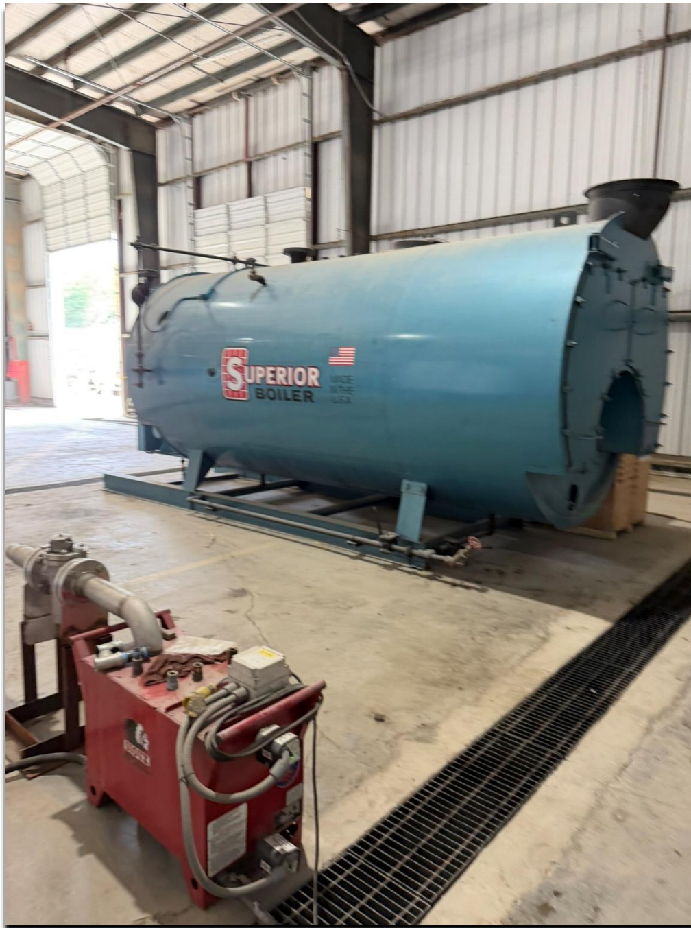
Photo 4 – Tank Wash Area (Boiler)
