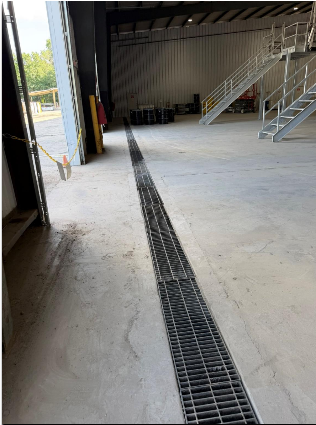
Photo 2 – Tank Wash Secondary Containment (Trench Drain)
